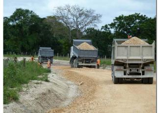
Camions carrying coral, 1, 2 & 3. The first one has spread its load, the middle one is about to and the rear one is waiting to. Currently 12 trucks are engaged in carting aggregate to the work site.
